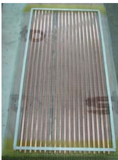
Fig. 6. Reinforced plaster board with horizontal gaps, arrangement of the reinforcement and of the formwork for the making of the horizontal gaps
