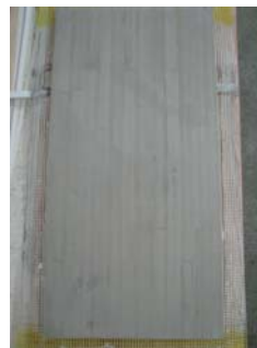
Fig. 7. Reinforced plaster board with horizontal gaps after the pouring of the densified plaster
