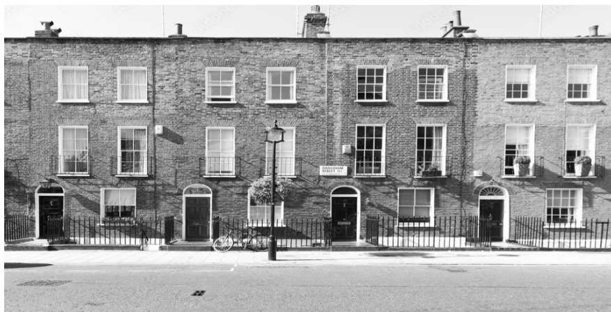
Fig. 1. Victorian terraced houses that have been restored [ https://as1.ftcdn.net/v2/jpg/02/23/33/38/1000_F_223333848_HpEsoczcaiMC2Cgh7GN3LaLExdNSbl2i.jpg ] (open source)
